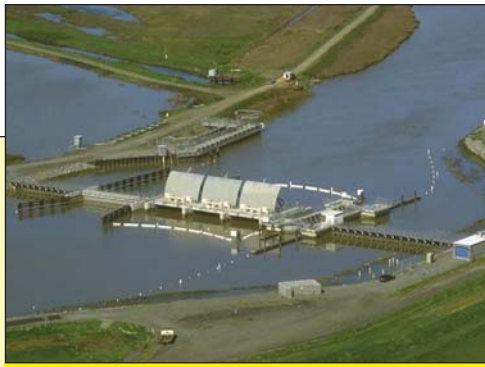
Gates designed to help manage salinity and tides already exist in the San Francisco Bay-Delta Estuary, such as these built in 1988 in Suisun Marsh to freshen the marsh for waterfowl habitat.
